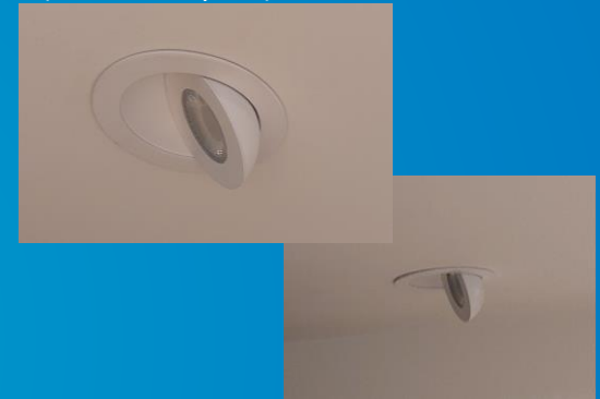
Highlight Ceiling LEDs (dimmable pots)
